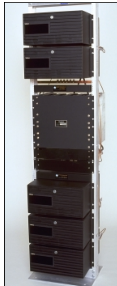
Five Channels and 7-Foot Rack
